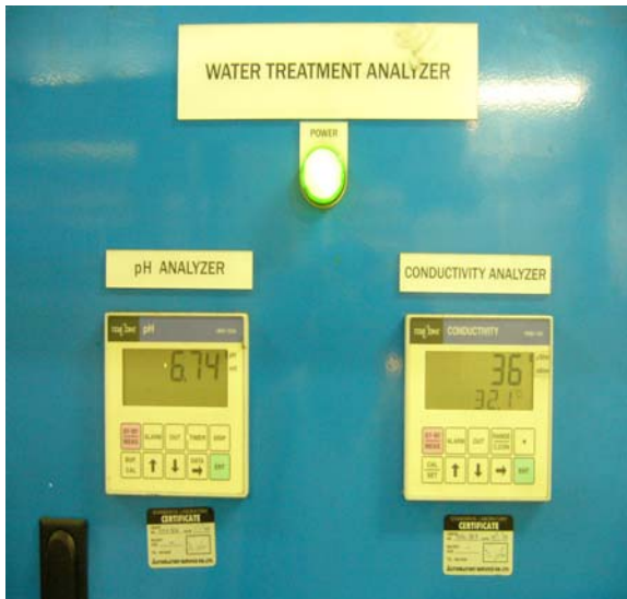
C-1 Cool water analysis at Area-2 pH = 6.74 , Temperature = 32.1oC Conductivity = 36.1 μscm
