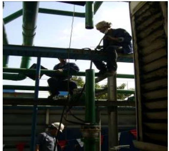
B-4 The pipe was cut above the pump 2.00 meters
