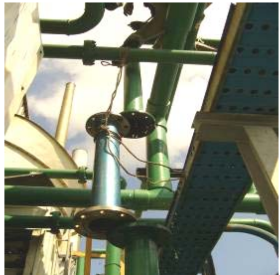
C-2 Removed CAT-100 after installed 60 days
