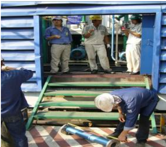
B-3 Reconfirm every things before cut the pipe
